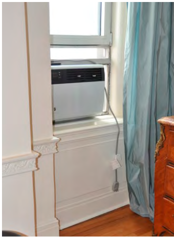
DINING ROOM -Plexi-glass seal around AC unit
