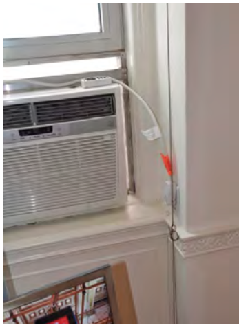
RECEPTION ROOM -Plexi-glass seal around AC unit
